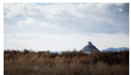
Deponie Rautenweg, Wien | AT
